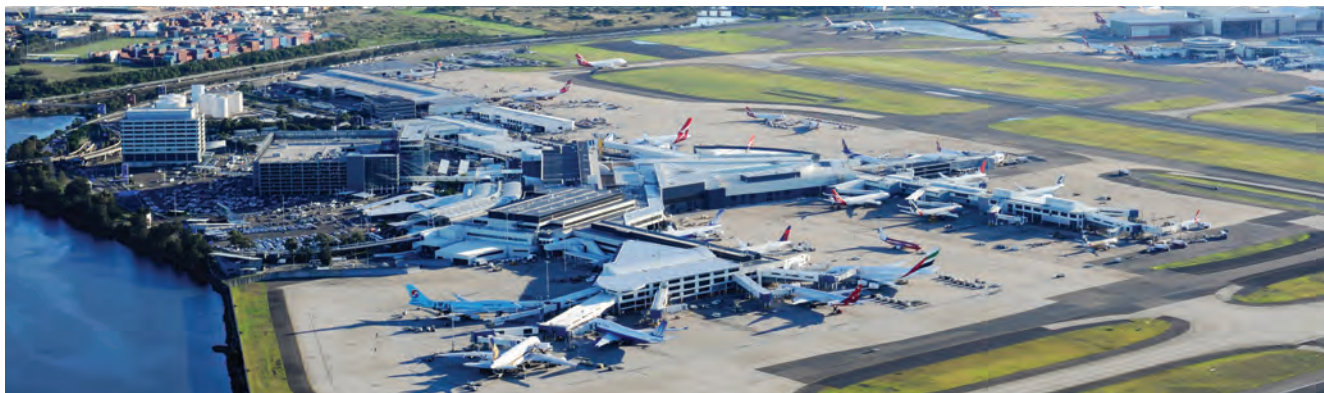
© 2016 State of NSW Transport for NSW.
