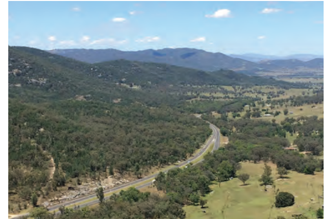
New England Highway looking South. © 2016 State of NSW Transport for NSW.
