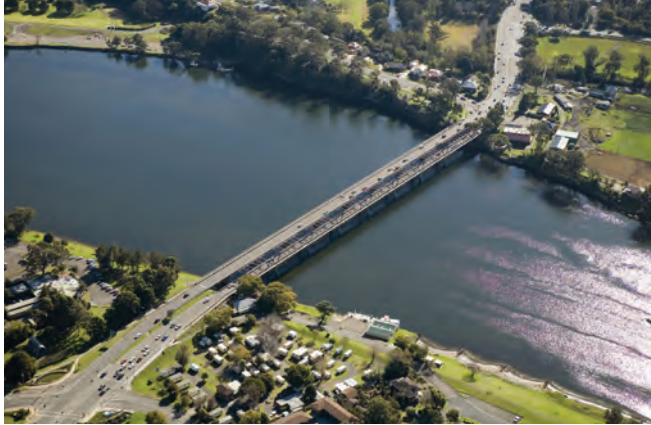
Nowra Bridge. © 2016 State of NSW Transport for NSW.
