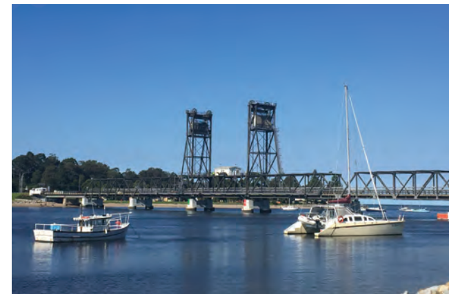
Batemans Bay Bridge. © 2016 State of NSW Transport for NSW.
